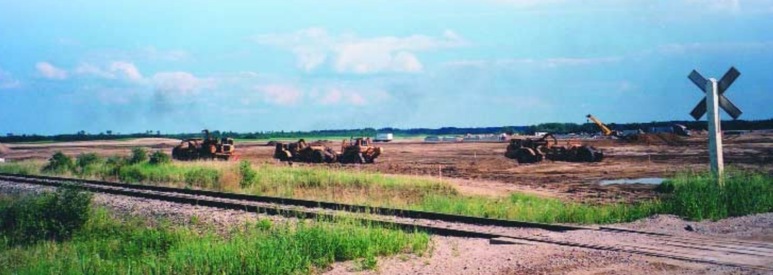
Early site work at Meadow Lake OSB.
