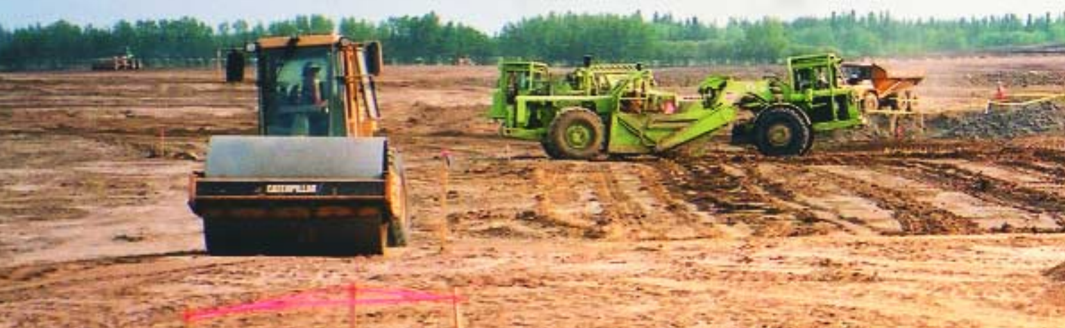
Site preparation at Meadow Lake OSB.
